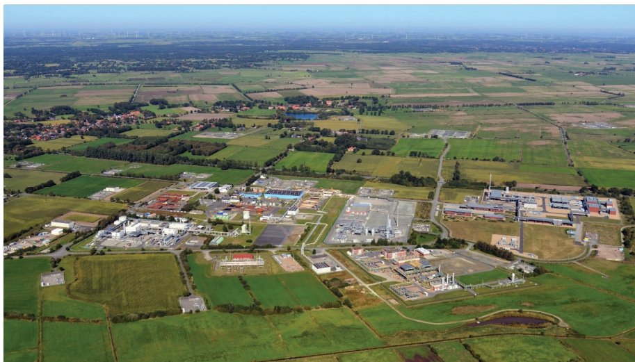
Fig. 1 Etzel Cavern Storage in recent days – Security of Supply with Natural Gas and Oil
